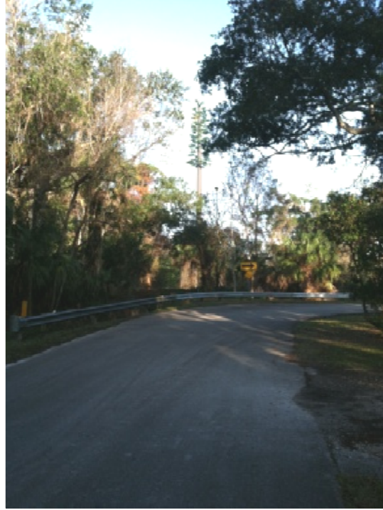
Looking N from residential area
