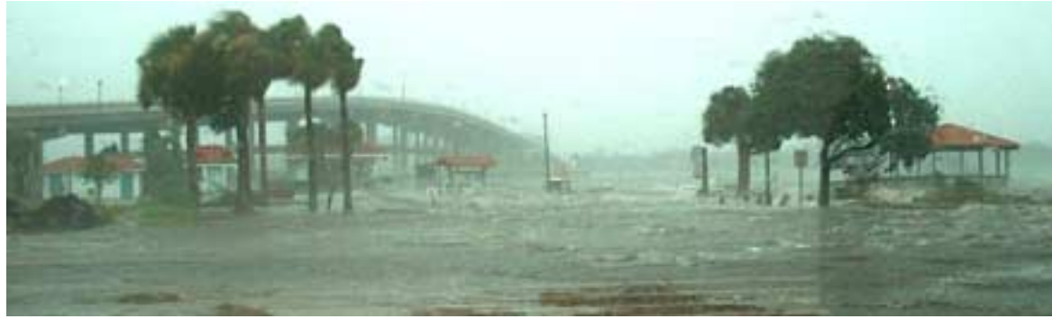
The fury of Hurricane Frances pushed the Halifax River over its banks at Cassen Park and the Granada Pier Bait & Tackle shop along Beach St. directly across from City Hall. The fishing piers and the bait shop survived the storm and are open again to the public. Photo by Ormond Beach Police.
